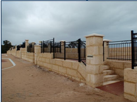
Reconstituted Limestone Retaining Wall
