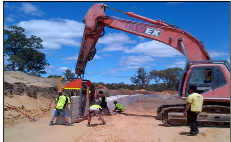
Wall Panel Installation
