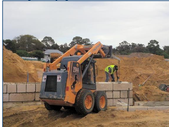
Retaining Wall Laying
